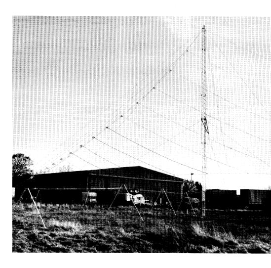
Only two sets of guys are required. There are no locking latches, sliding sections or elaborate cable and pulley arrangements to malfunction; the design simplicity increases ease of assembly and reliability.
