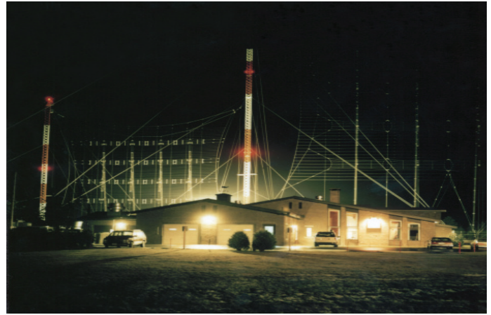
Figure 1. Take-Off Angle – Dipole Curtain Array with reflecting screen
